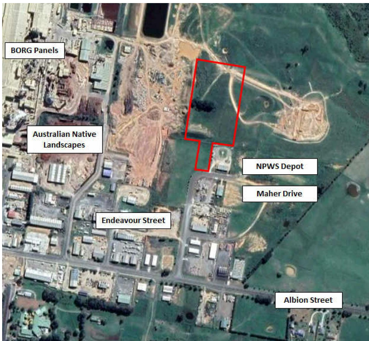
Figure 3: The subject site locality and context.
